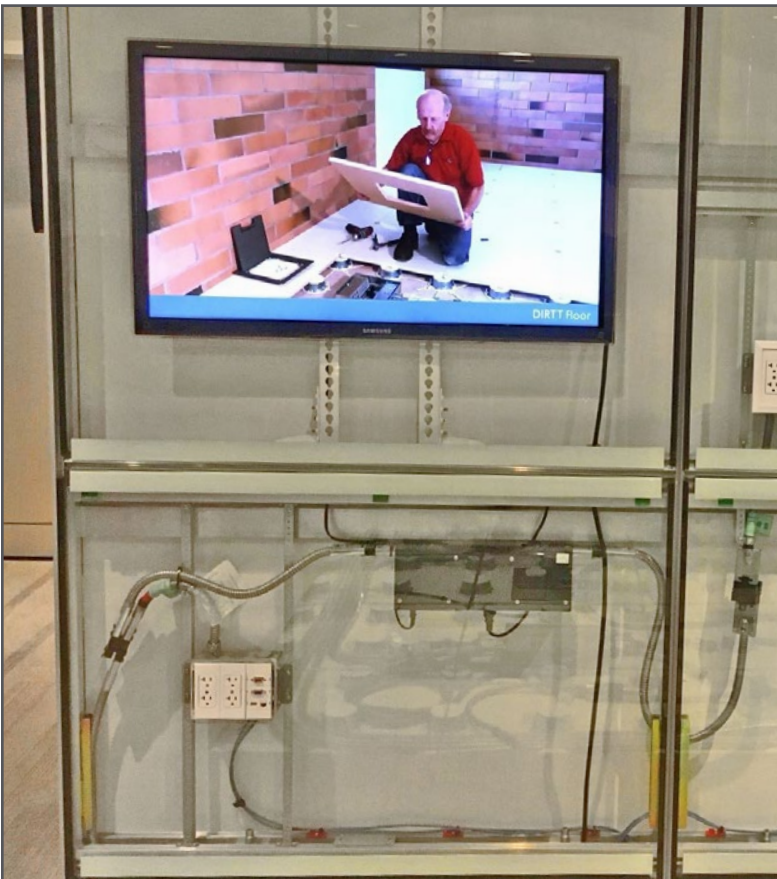
Figure 2: Cable management in a DIRT wall.
